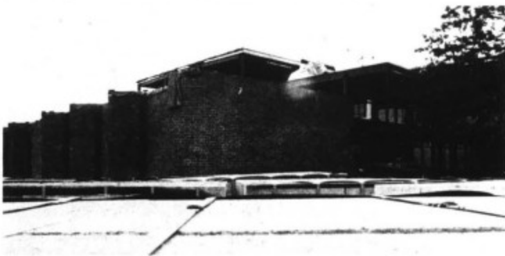
Work continues at a slow but constant pace on the newest addition to the Furman physical plant — the Daniel Music Building — now scheduled for completion this summer.
